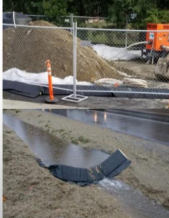
TRIANGULAR SILT DIKE
